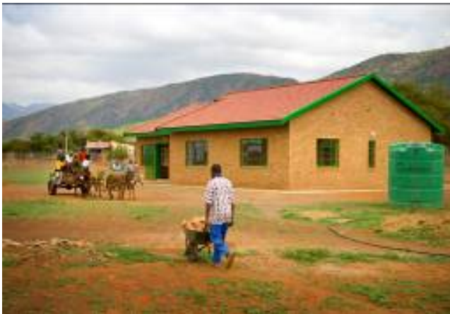
New clinic under construction - Lebowa
