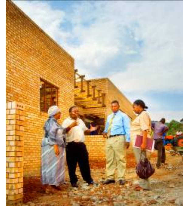
Lebowa – Bakery under construction
